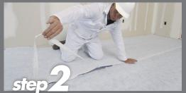
Seams between sections of sound mat are adhered with zip-strips or taped.\*
