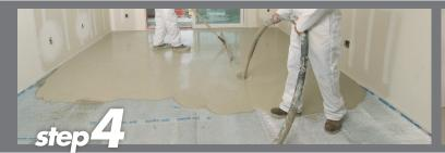
Sound mat is topped with an approved Maxxon Underlayment, at a depth<sup>†</sup> specific to the application. To ensure uniform depth and a smooth finish, installers use a screed to finish the underlayment surface. (If Acousti-Mat is installed only in hard surface areas, the underlayment is poured directly over the subfloor in areas to be covered with carpet and pad.)
