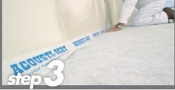
Isolation strips are installed, then taped, around the perimeter of the rooms receiving Acousti-Mat to eliminate flanking paths. Isolation strips are also installed, then taped, around any vertical penetration through the floor.
