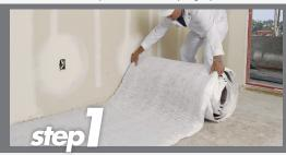
Sound mat is loose laid over the entire concrete or wood subfloor.
